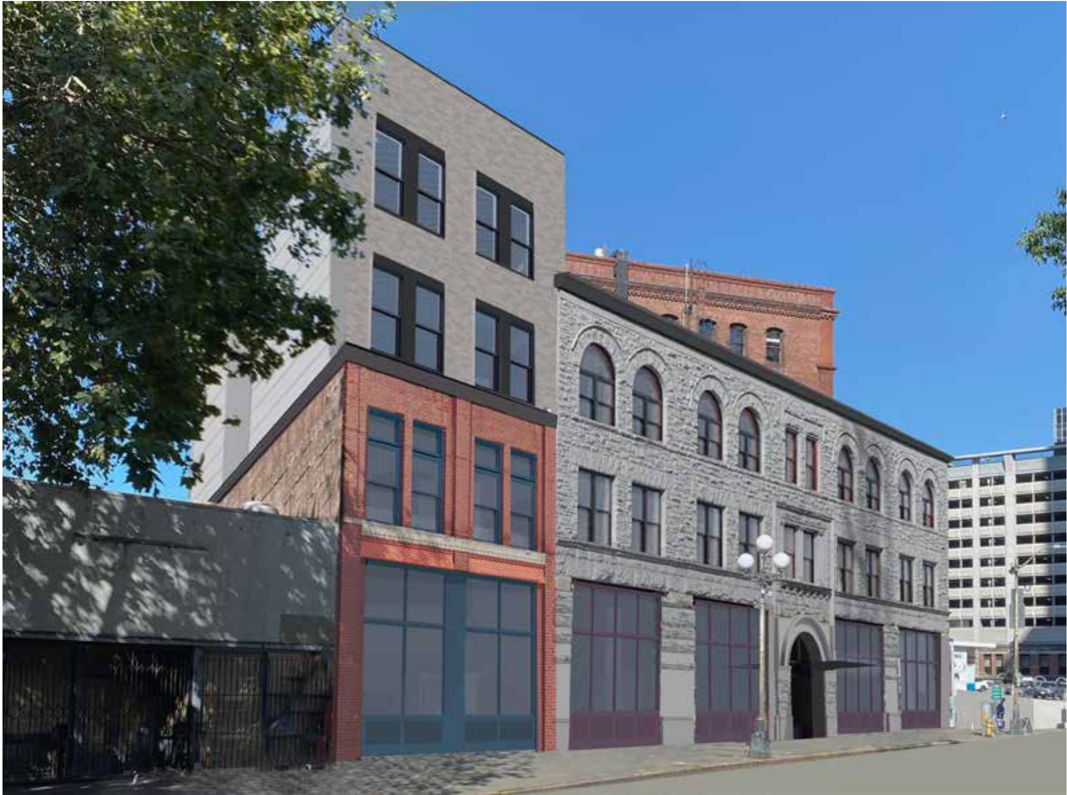
View looking north-west on Second Ave
